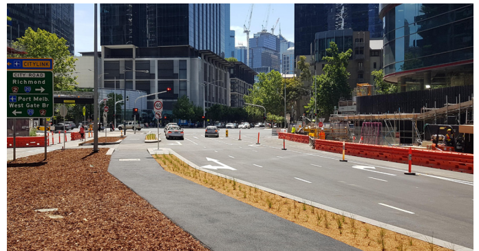
The roadway is now open between Kavanagh Street and City Road
